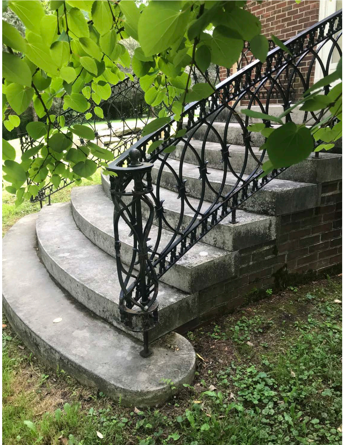
Wrought iron handrail at Mercygrove
